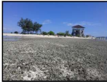
Figure 7. Coral gravel deposition formed by erosion in the southern part of the island.
